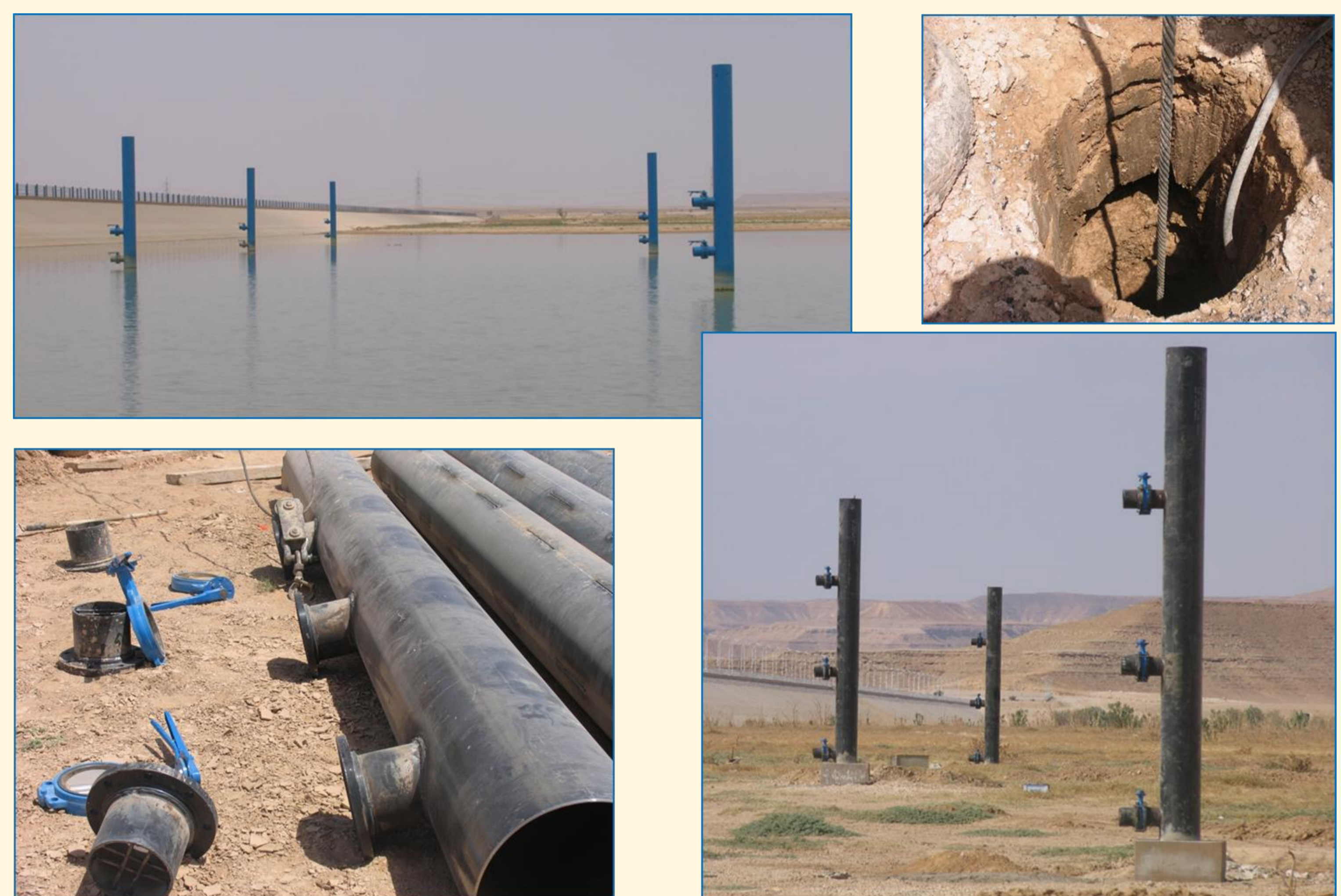
Fig. 3: Al-Alb dam next to Riyadh with infiltration wells [4].
