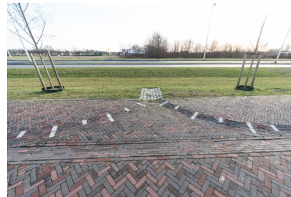
6 Gully free road to swale, Almelo
