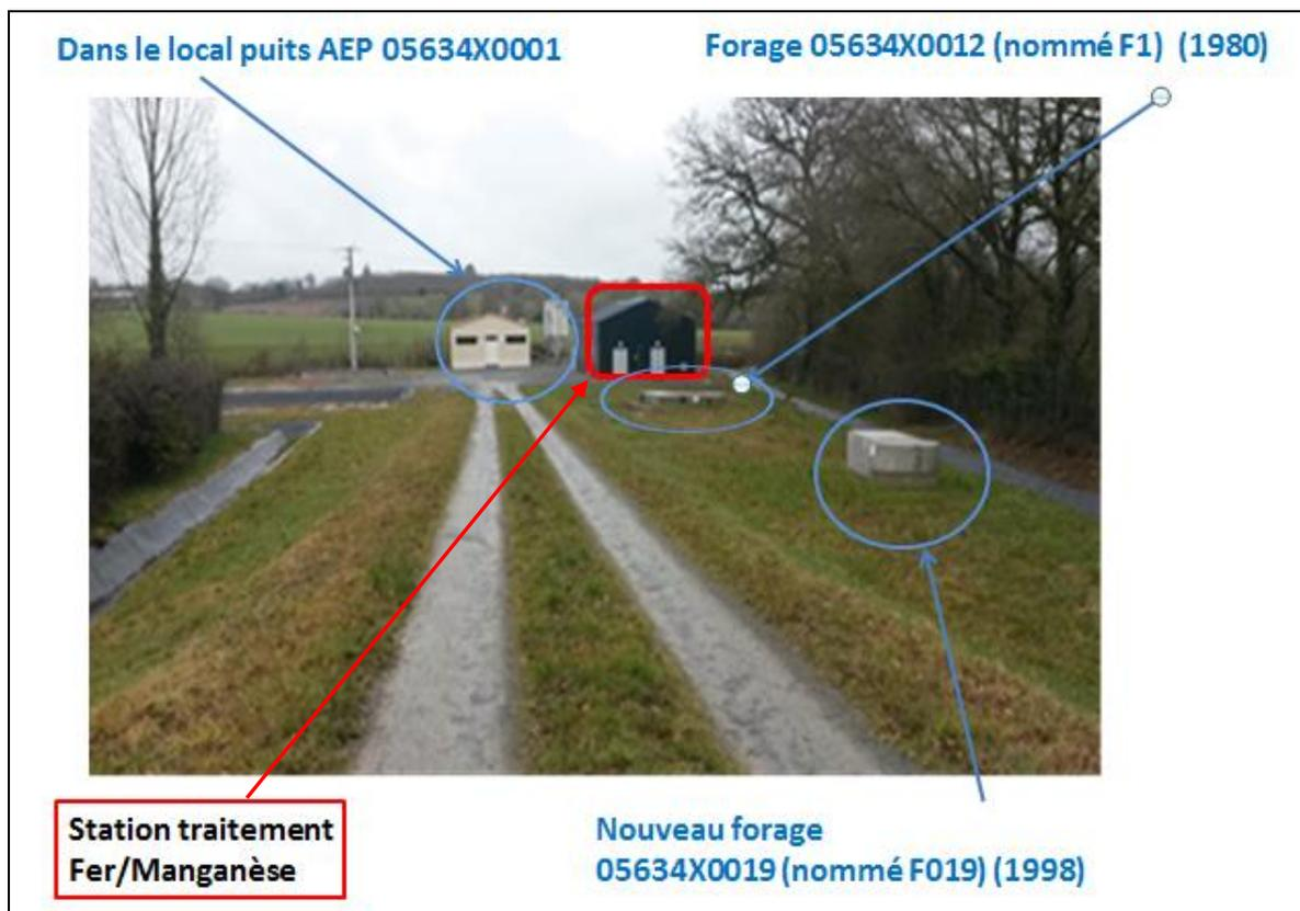
Figure 24 – View of the installation of drinking water supply, The Tail, Pouzauges
